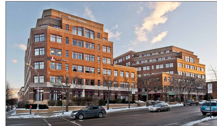
100 Middle Street , whose two towers contain 195,000 square feet, sold for $35 million to Portland Albany Road Real Estate Partners, a Boston-based firm. Greg Boulos and Joe Porta of CBRE|The Boulos Company represented the seller.
